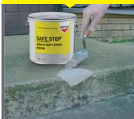
SAFE STEP® Heavy Duty Epoxy Repair
